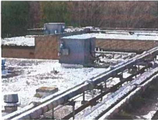
Figure 1 - Existing Magic Aire Rooftop Air Handlers
