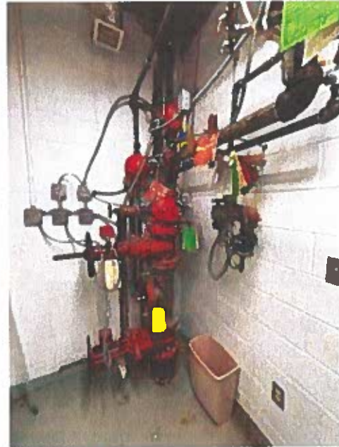
Figure 20 - Existing sprinkler riser for addition
