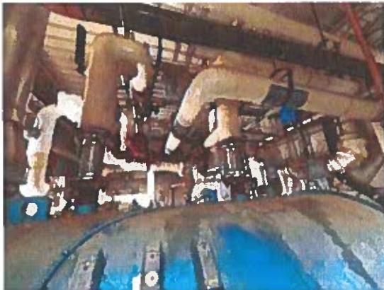
Figure 3 - Existing Superior Boiler and Hot Water Piping
