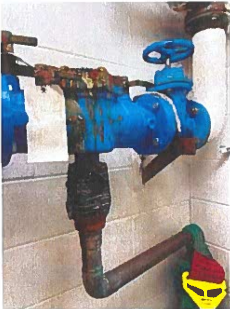
Figure 14 - Existing backflow preventer in addition addition
