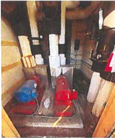
Figure 9 - Chilled water piping from district plant (right) and existing chilled water pumps (center)
