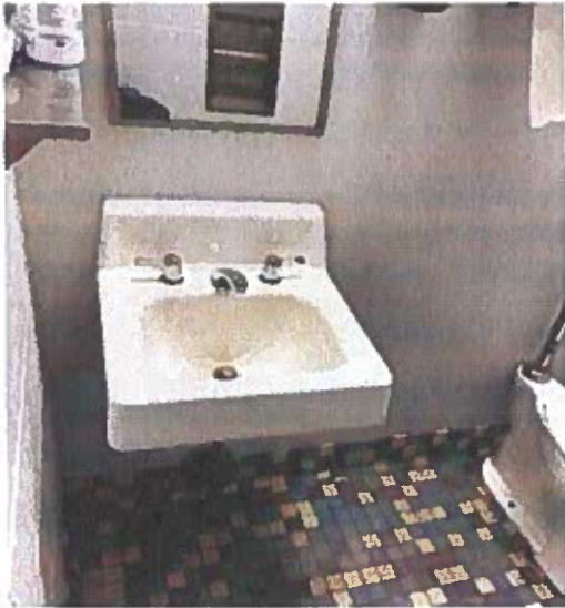
Figure 16 - Manual controls on sink fixture in cell
