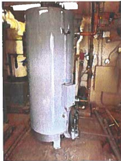
Figure 13 – Existing water heater for original building
