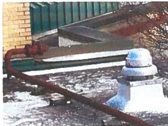
Figure 18 - Existing gas piping on roof
