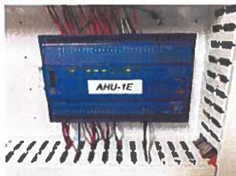
Figure 11 - Distech controller for AHU-1E
