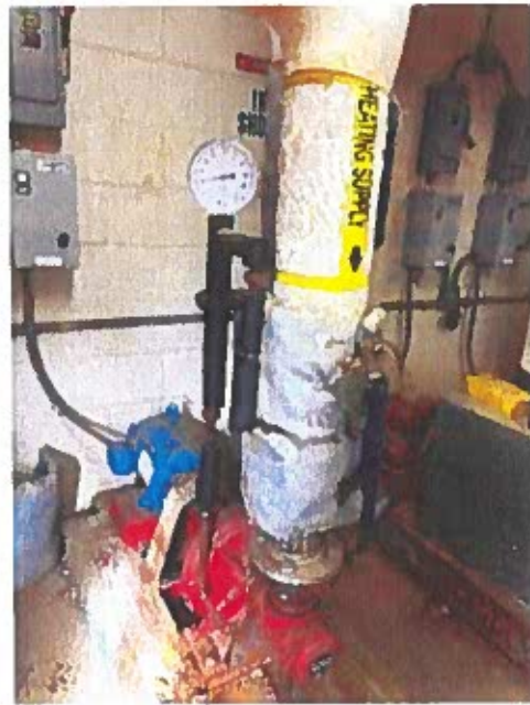
Figure 4 - Existing Hot Water Pump
