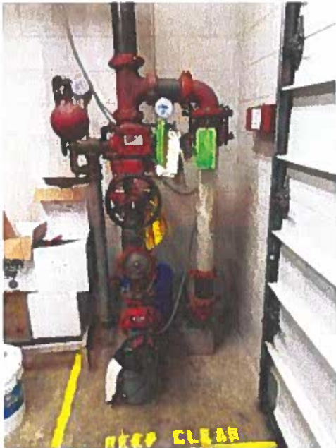
Figure 19 – Existing sprinkler riser for original building
